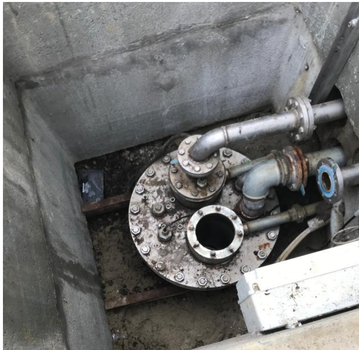
Example of Booster for two pumps
