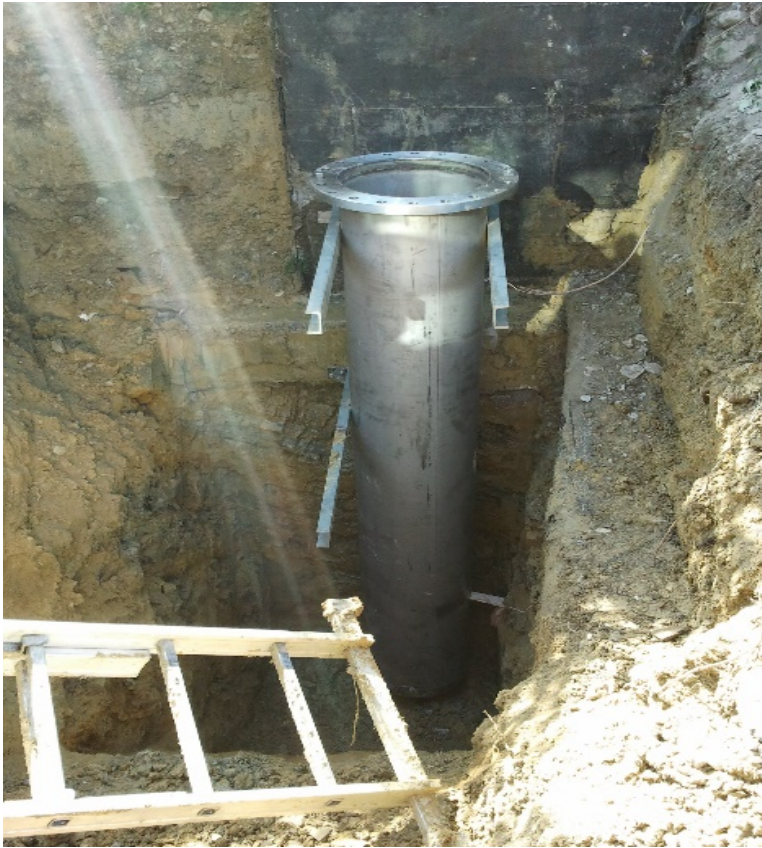
Positioning the booster in the ground adjacent to the tank
